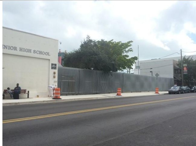
Site Facing NE 2 nd Avenue
