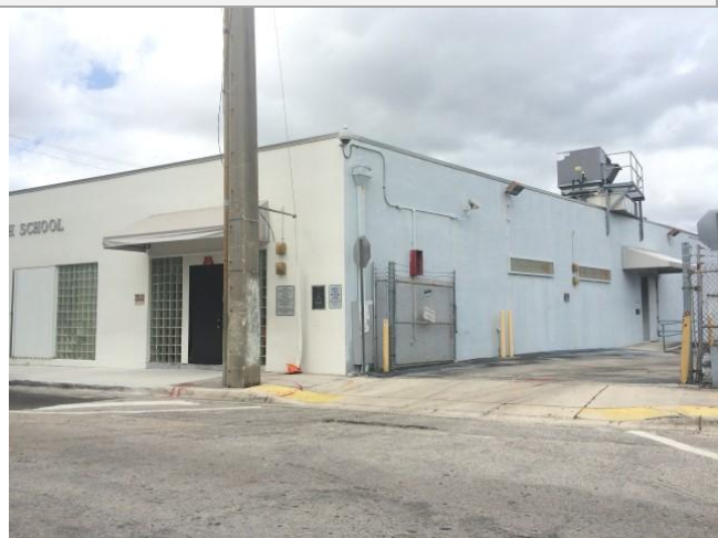
Improvements Facing NE 39 th Street
