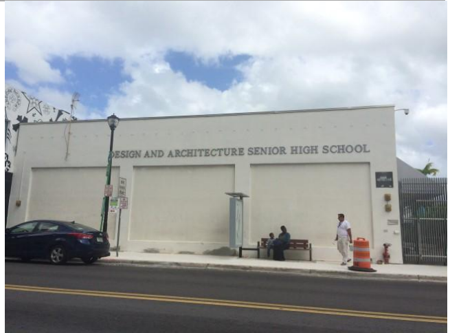
Site Facing NE 2 nd Avenue
