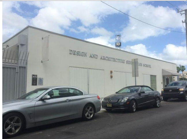
Site Facing NE 2 nd Avenue
